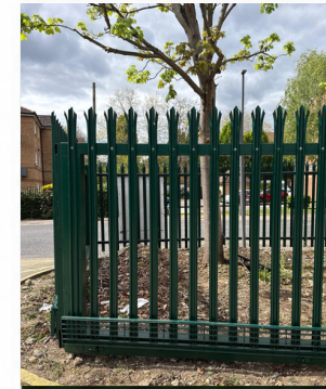
Upgraded fencing installation
