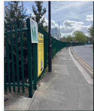
New secure perimeter fencing
